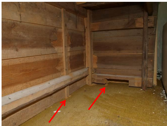
Fig. 8. Bore dust inside the altar
