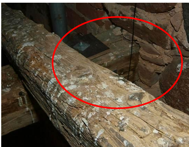
Fig. 7. Load-bearing timber element is uninsulated with hydro-insulation - stonewall damps the timber, which may result in the reduction of shear strength
