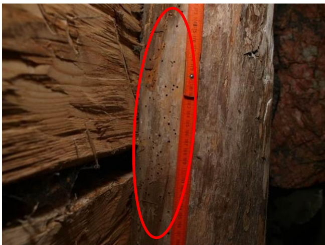
Fig. 10. Damaged underground floorbeam
