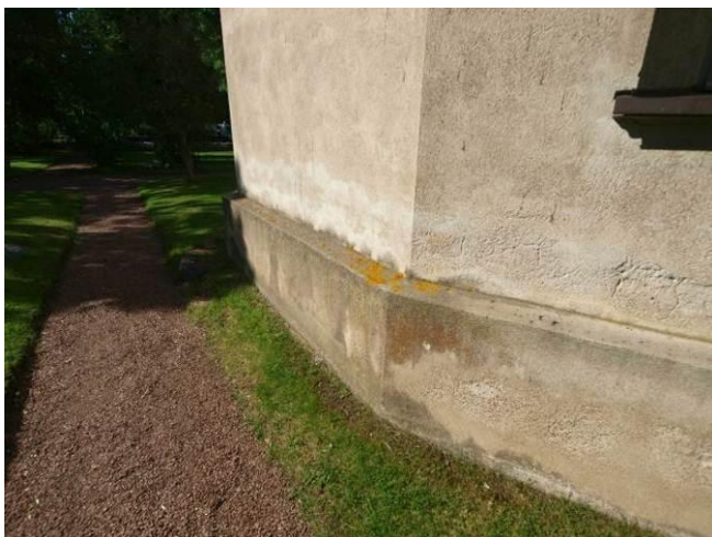
Fig. 3. The outreaching part of the wall is bio- and moisture damaged
