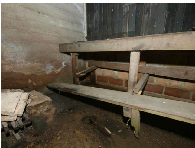
Fig. 13. Degraded timber elements in sauna
