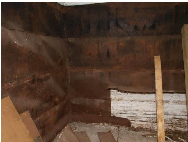
Fig. 12. Sheet metal covered walls in room No. 8
