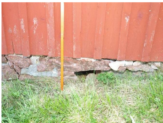
Fig. 2. Loose or missing mortar between quarry stones of the socket
