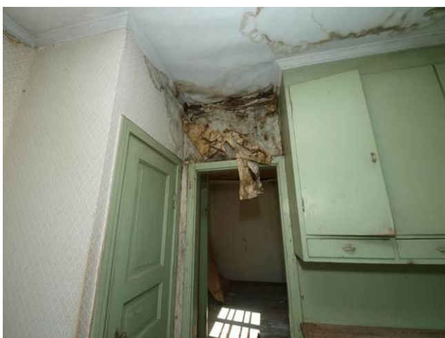
Fig. 21. Severe water damages in the kitchen
