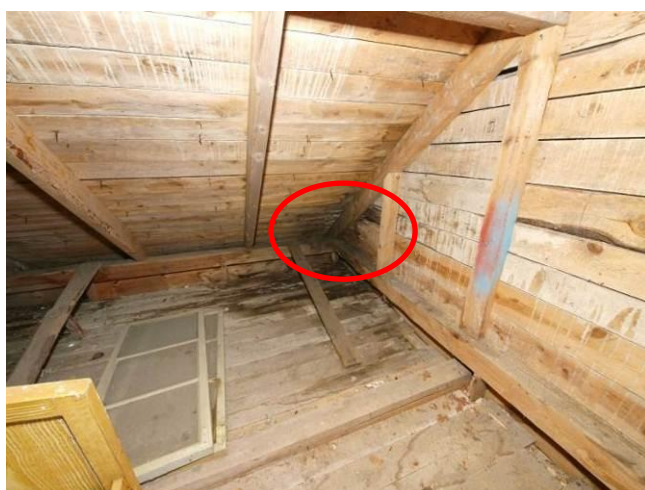
Fig. 39. Beetle damages on the roof's timber structure and fungal damage on the floorboards
