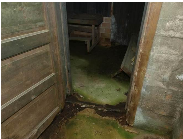
Fig. 10. The basement's floor is covered with algae and the timber elements are degraded
