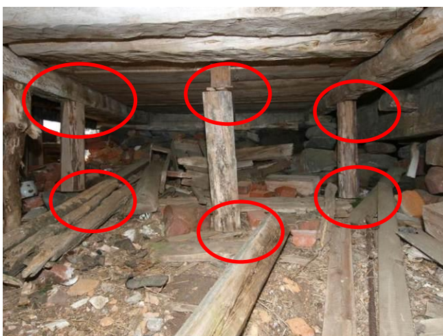
Fig. 4. The load-bearing posts are not firmly set to the ground and joined to the floorbeams, also direct moisture contact from the ground
