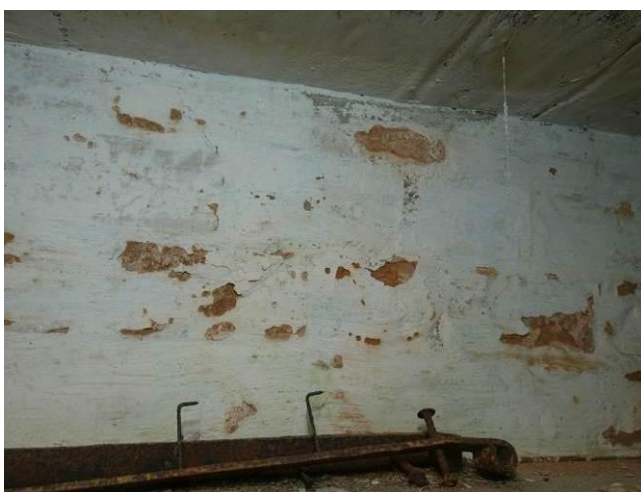
Fig. 15. Moisture- and frost damage causing plaster to flake off
