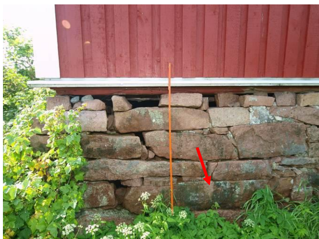
Fig.2. Piled socket partly without any mortar, biodamage on the socket
