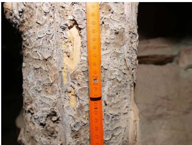
Fig.15. Bark beetle attacks in the cellar
