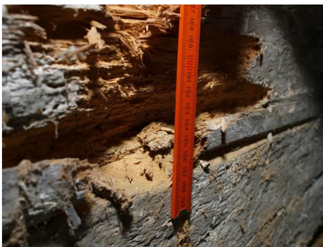
Fig. 15. Insect damages on the wall of room No. 4.
