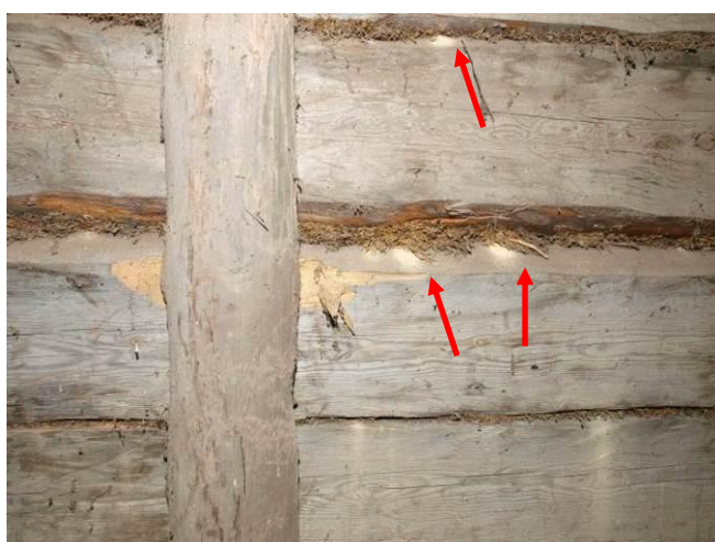
Fig. 13. Bore dust in the attic wall
