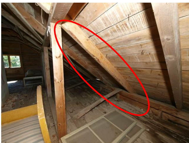
Fig. 35. Longhorn beetle ( Callidium violaceum ) damage on roof's timber structure
