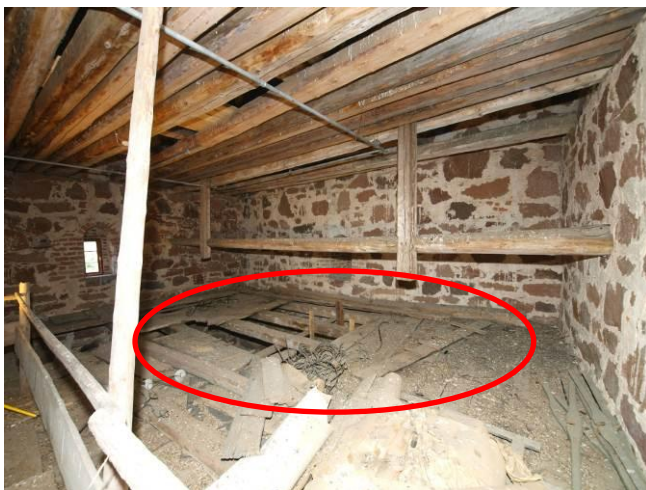
Fig. 5. The whole floor is covered with birds' excrements and some elements of the timber floor are damaged
