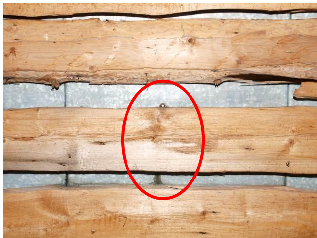
Fig. 7. Water passage in the metal roofing
