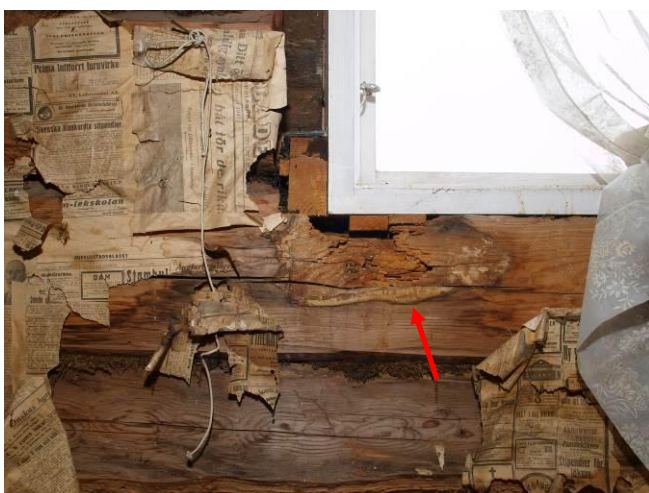
Fig. 17. Old fungal damages on the wall under window in the room No. 15
