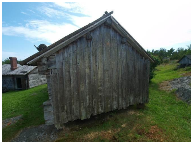
Fig. 3. Lichens have covered the shed exterior wall panelling
