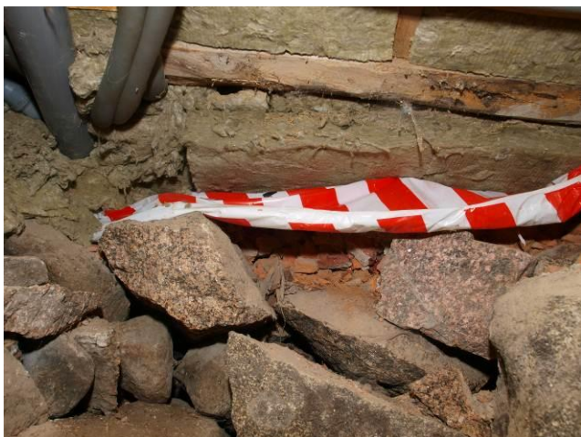
Fig. 6. Uncovered thermal insulation (in the basement)
