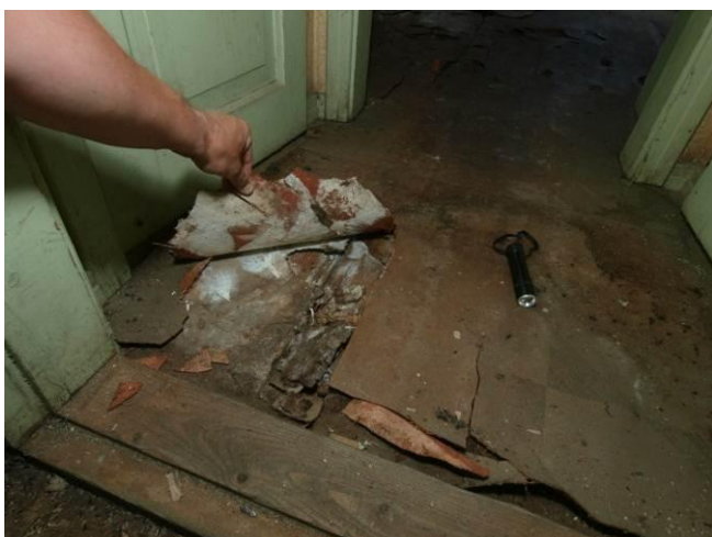
Fig.33. Mycelium of Antrodia on the floor material in the hall
