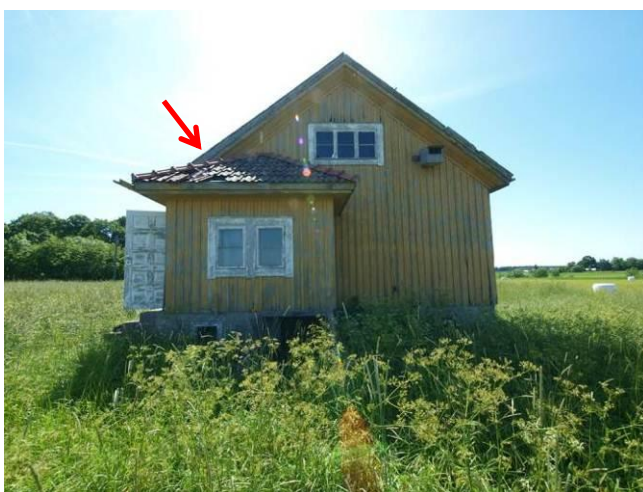
Fig. 8. Some roofing tiles are missing and broken on the northern side
