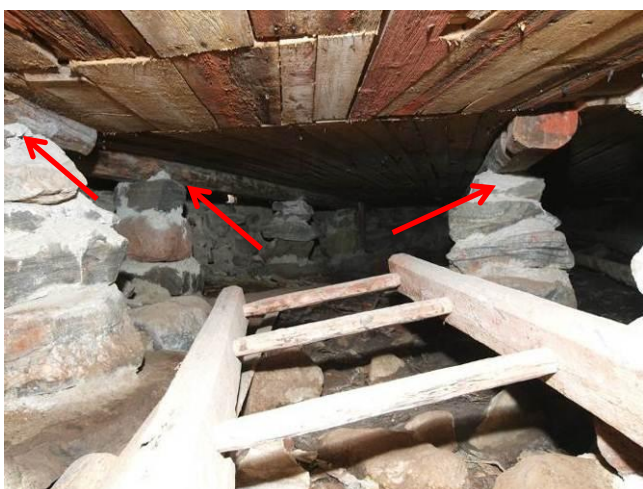
Fig. 4. Missing hydro-insulation between the bearing floorbeams and stone foundation
