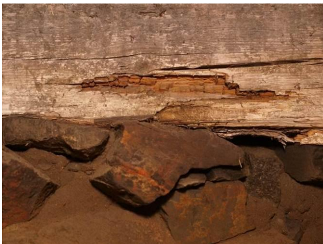
Fig. 5. Missing hydro-insulation between the bearing floorbeams and stone foundation
