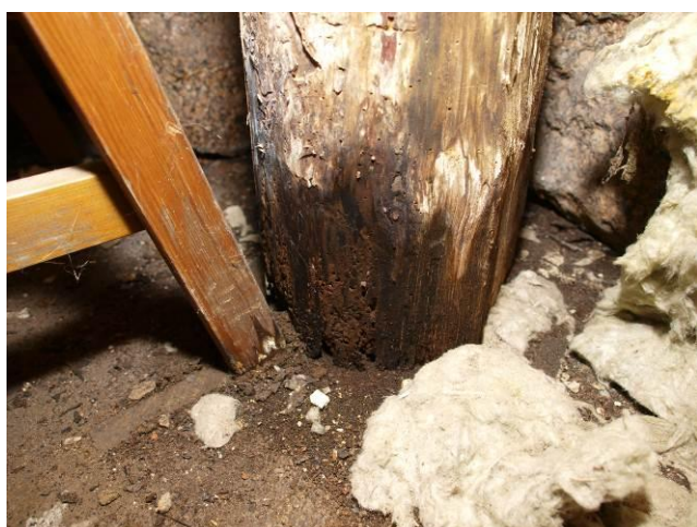
Fig. 4. Missing hydro-insulation, anobiidae beetles damage (in the basement)
