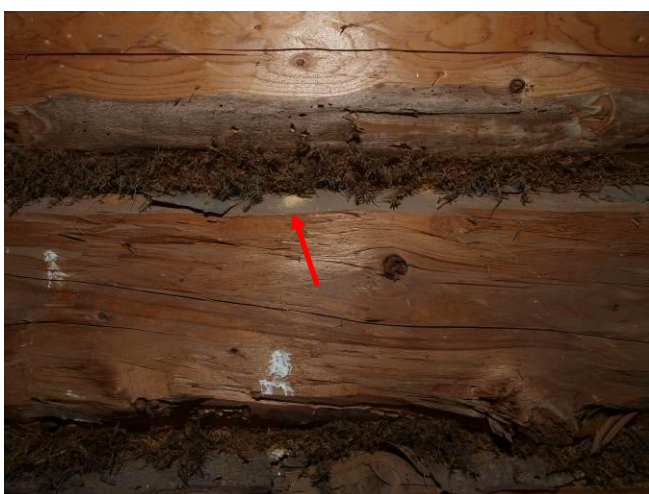
Fig. 19. Exit holes and bore dust on the wall in the attic
