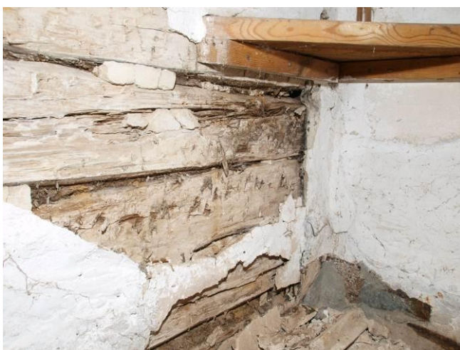
Fig. 9. Loose and missing plaster on the wall in room No. 6
