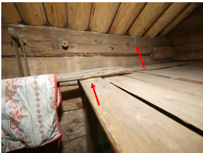
Fig. 5. Bore dust under the timber bar and on the upper part of the walls
