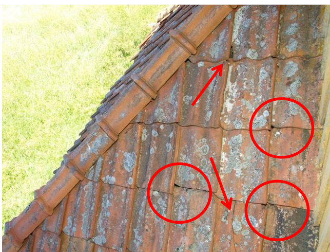
Fig. 30. Many of the rooftiles are broken and covered with lichens
