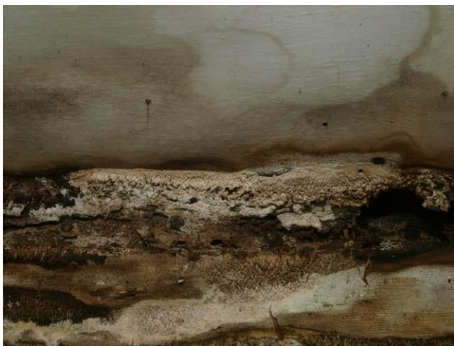
Fig. 34. Fruitbody of Antrodia species on the floorbeam
