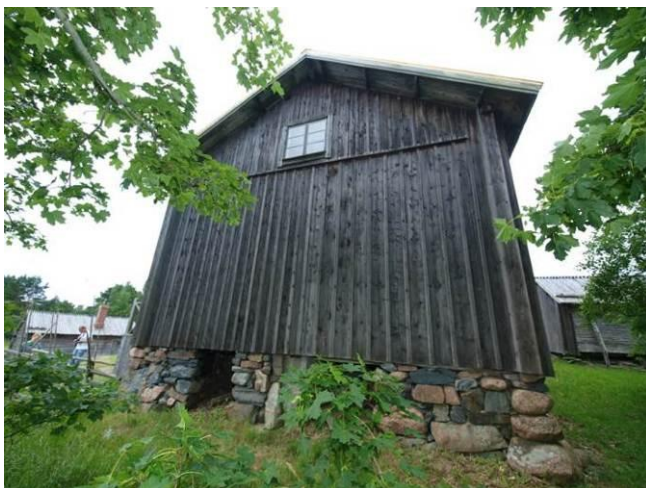
Fig. 3. The socket is piled mostly without any mortar
