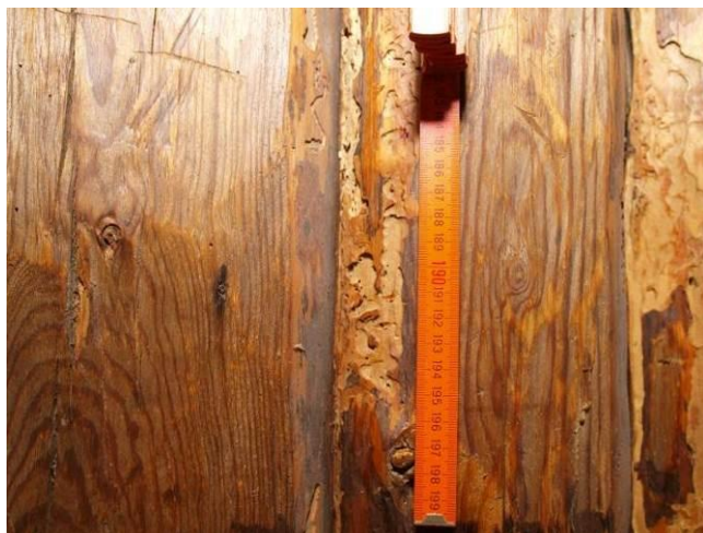
Fig. 13. Larvae tunnels on the surface of timber made by bark beetles
