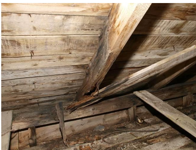
Fig. 29. Due to the water leakage, the rafter and the wind beam has degraded and lost its strength
