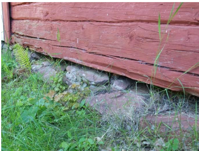
Fig. 3. Missing quarrystones in the socket
