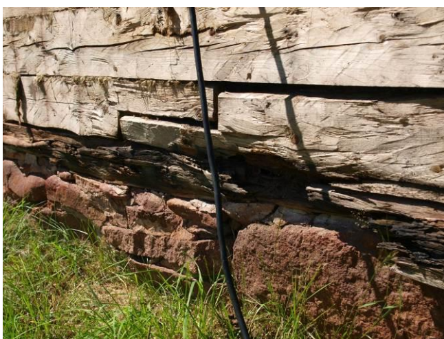
Fig. 4. There is a lack of hydro-insulation between the logs and quarrystoned socket
