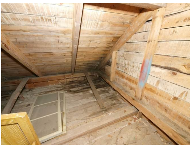
Fig. 27. Waterdamage in the attic's northwest corner
