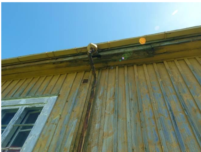
Fig. 3. Corroded and malfunctioning rainwater pipe
