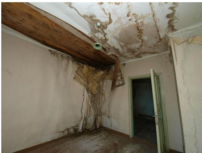
Fig. 22. Severe water damages in the livingroom
