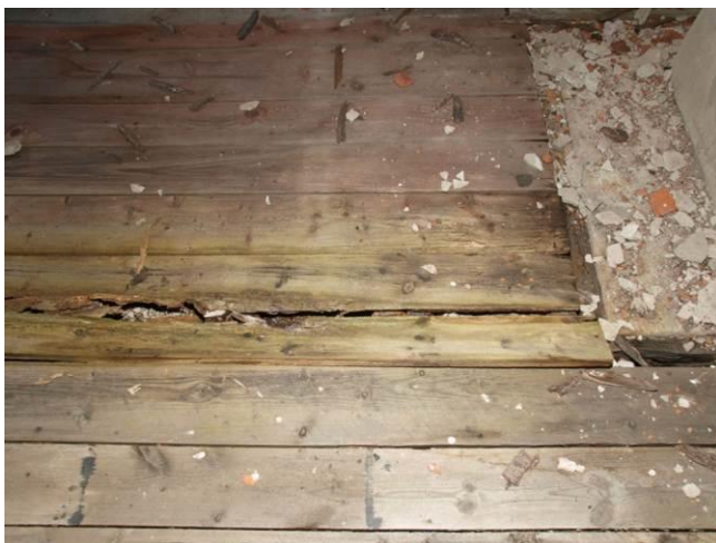
Fig. 28. Severe water damages in the attic's floor
