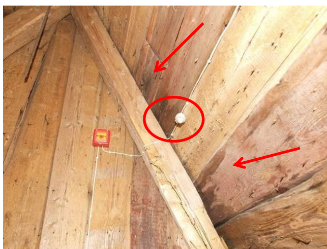
Fig. 9. Roof boarding has marks of water passages and wasp's nest
