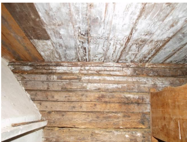
Fig. 4. Traces of water passages in room No. 3
