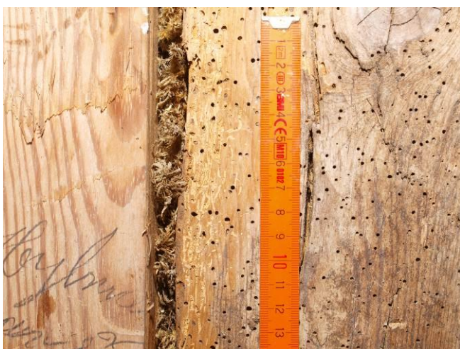
Fig. 20. Exit holes on the wall in the attic
