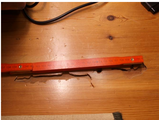
Fig. 11. Damages by the Old House Borer in the living room floor
