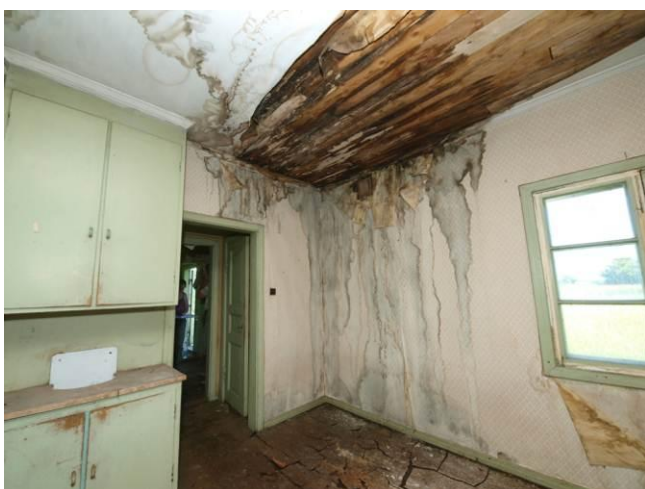
Fig. 20. Severe water damage in the kitchen
