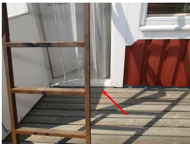
Fig. 7. The balcony's floor should be lower than the floor inside the building
