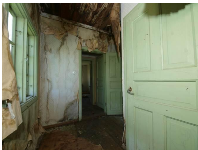
Fig. 18. Severe water damages in the hall room
