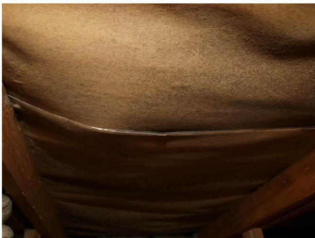
Fig. 12. Moulds on the the surface of the roof boarding
