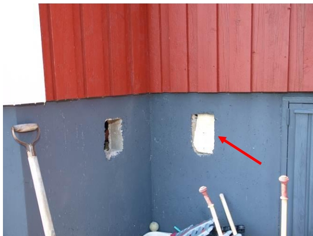
Fig. 2. Closed ventilation hole
