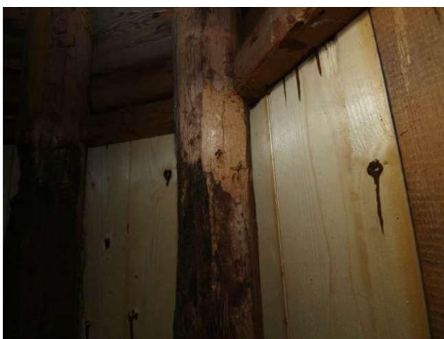
Fig. 7. Diagonal corner post with mechanical damages
