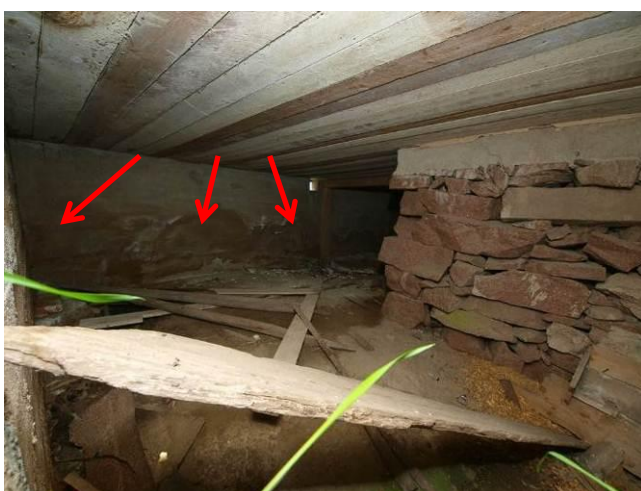
Fig. 16. Moisture and salt damages on the walls of the southern part of the basement
