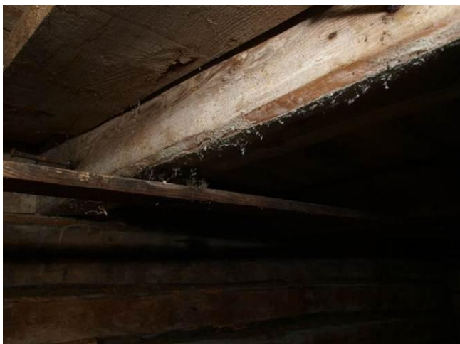
Fig. 11. Salt damaged ceiling-beam in room No. 2
