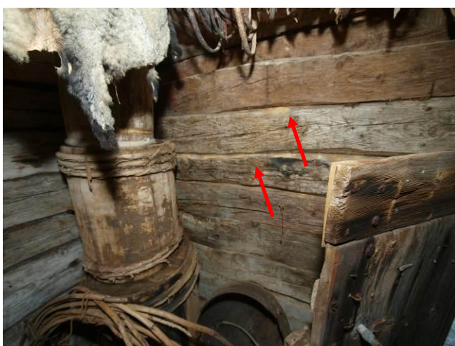
Fig. 6. Bore dust on the inside wall of the shed
