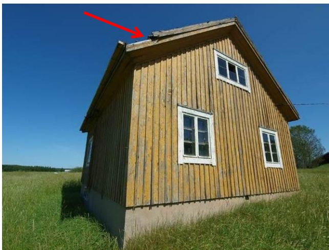
Fig. 6. Missing eave-boardings, paint has flaked off
