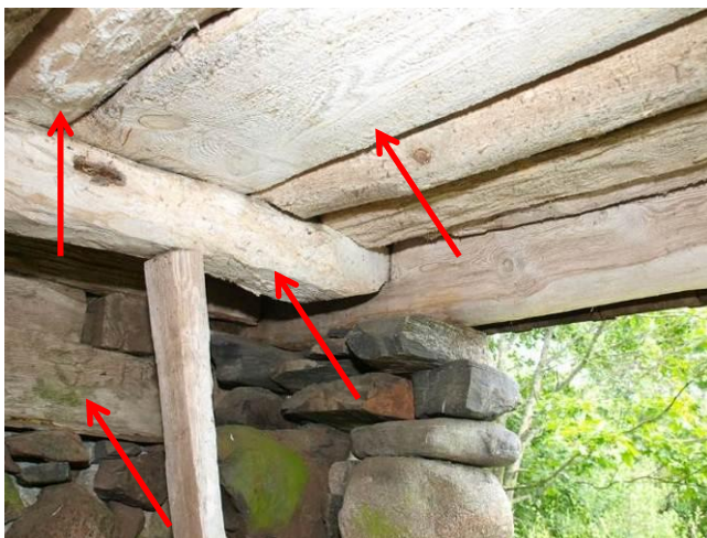
Fig. 8. Salt and biodamages on the floorboards and –beams
