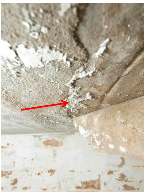
Fig. 12. Salt damages in the ceiling
