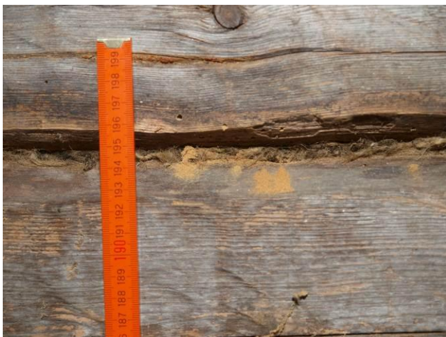
Fig. 6. Bore dust on the damaged wall in the room No. 1
