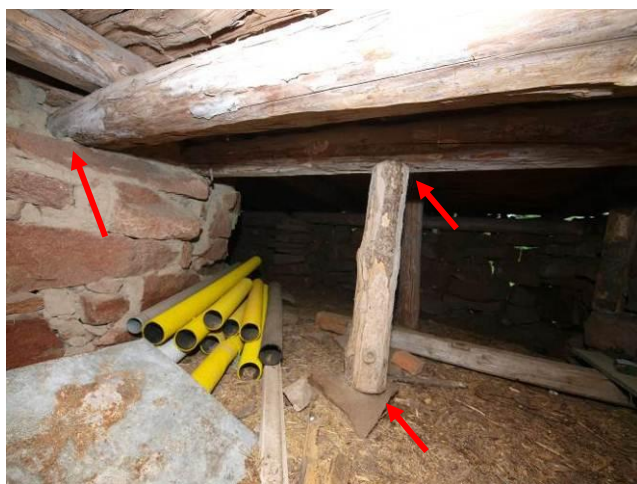
Fig. 3. Missing hydro-insulation, unstable timber joints
