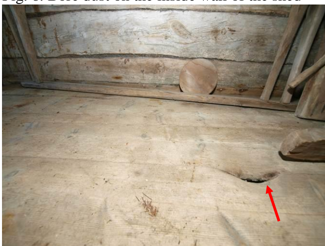
Fig.7. Hole in the floor made by rodents
