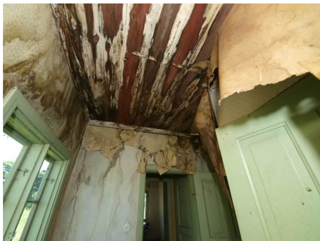
Fig. 17. Severe water damages in the hall room
