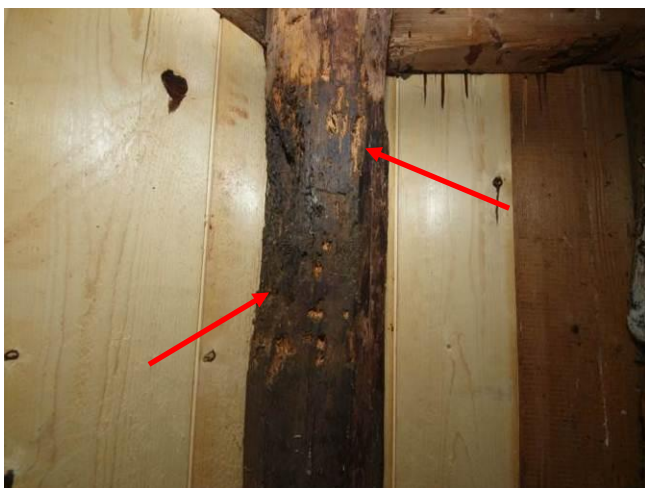
Fig. 6. Diagonal corner post with mechanical damages
