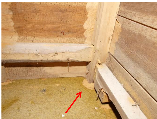
Fig. 9. Closer view to the bore dust inside the altar
