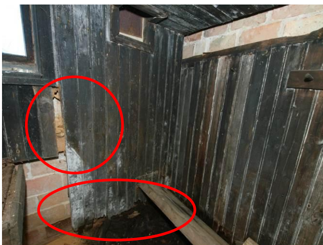
Fig. 31. Beetle attack on the timber of sauna wall
