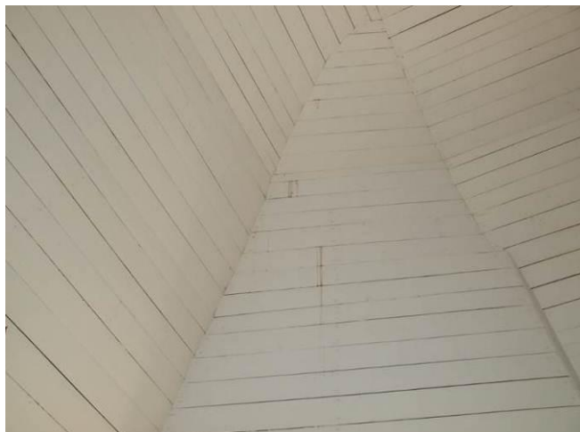
Fig. 8. Traces of water passage on the eastern part of the ceiling in the hall room
