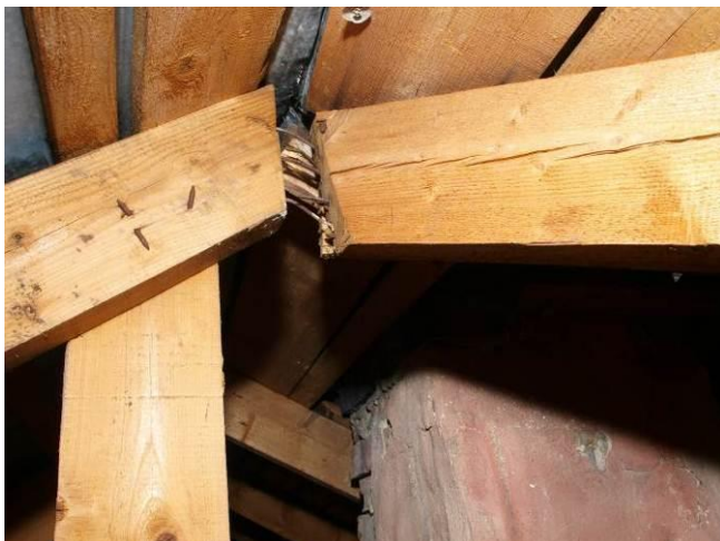
Fig. 14. A loose connection of the roof's timber structure
