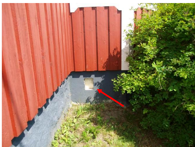
Fig. 3. Closed ventilation hole
