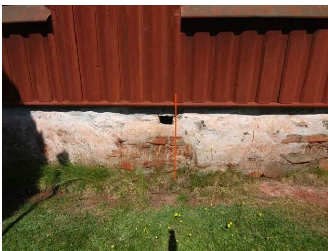
Fig. 3. There is some loose and missing plaster on the socket
