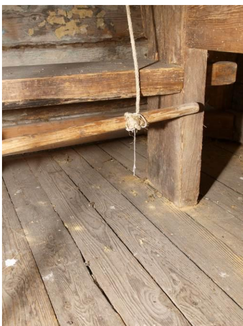
Fig. 8. Handlooms attacked by furniture beetle
