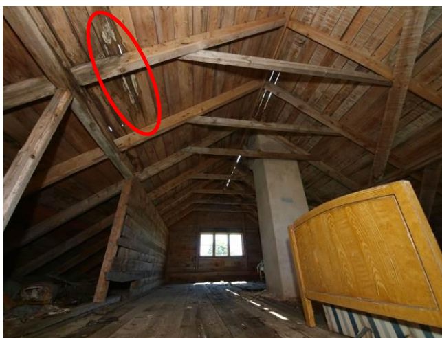
Fig. 36. Fruitbodies of Corticiaceae species on the roof's timber structure
