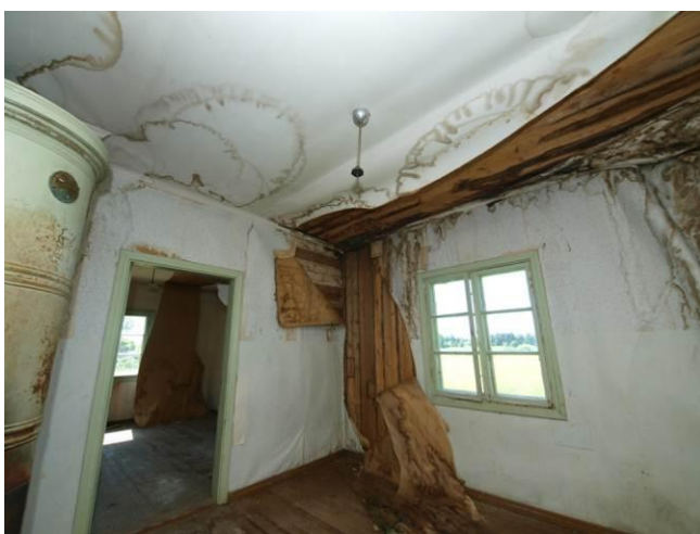
Fig. 23. Severe water damages in the livingroom
