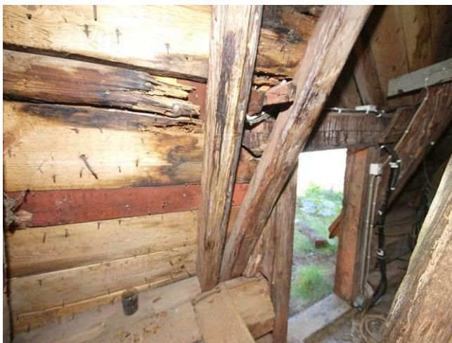
Fig. 3. Degraded diagonal posts and roof's timber boarding near the entrance
