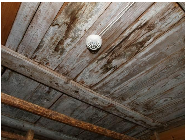
Fig. 5. Traces of water passages in room No. 4
