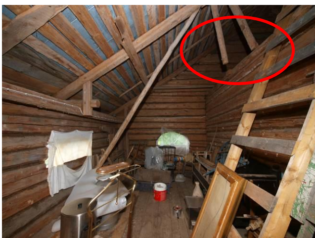
Fig. 12. Detached timber element
