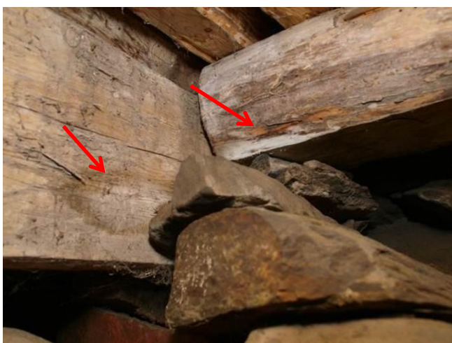
Fig. 7. Missing hydro-insulation and damped areas on floorbeams and foundation. Bio damages are on the floorbeam
