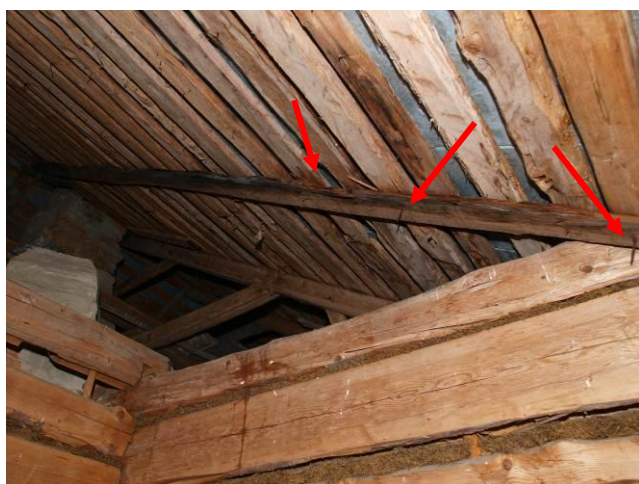
Fig. 8. Traces of water passages, caused by the nails, that are striked through the metal sheet roofings
