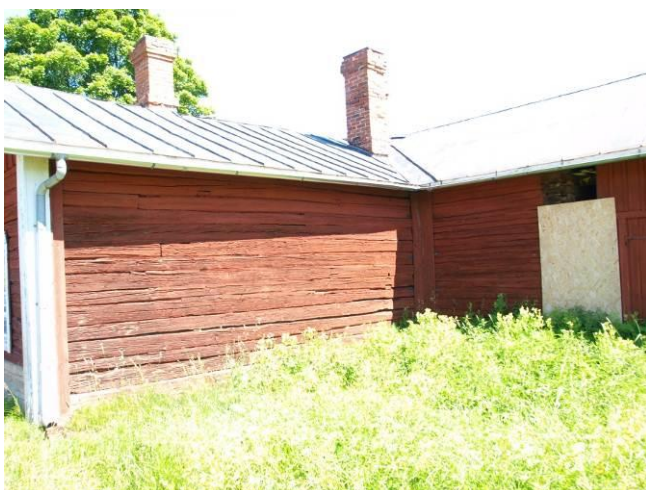
Fig. 7. The southern side of logwalls have severe UV-damaged
