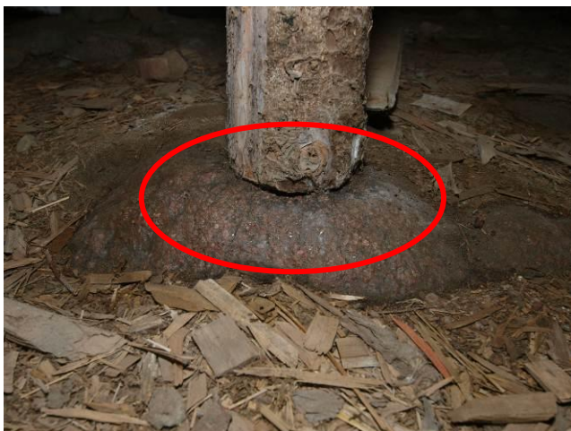
Fig. 5. Missing hydro-insulation
