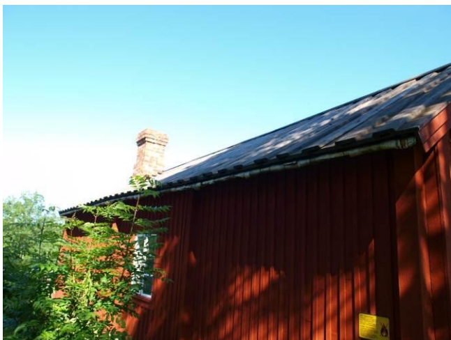
Fig. 3. The southern roof side undulates, which indicates deformations of the load-bearing structures
