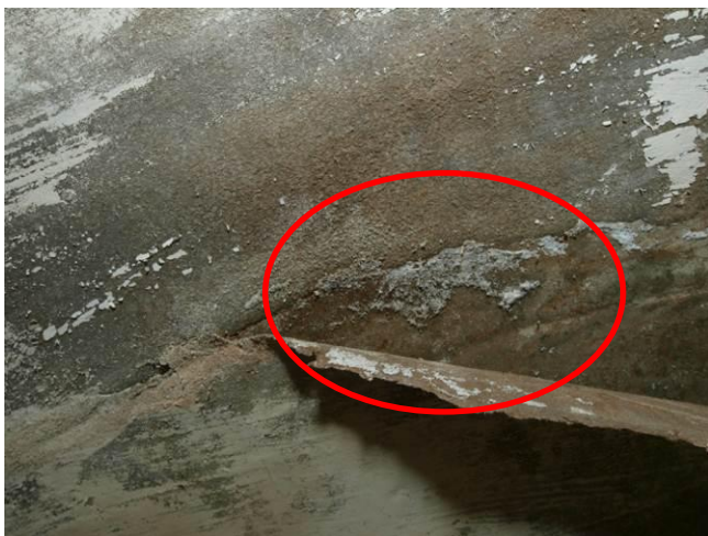
Fig. 11. Salt damages in the ceiling
