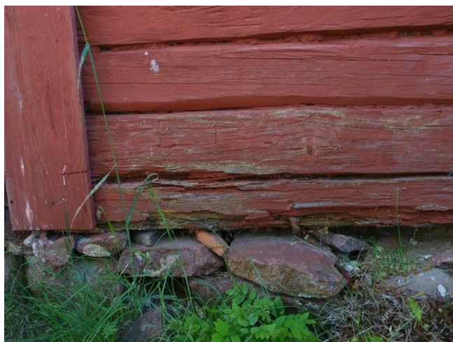
Fig. 2. Loose and missing mortar between quarrystones of the socket
