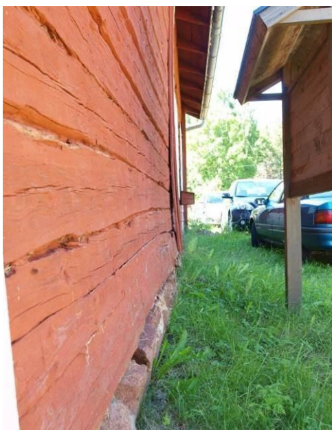
Fig. 5. Wall slanted out
