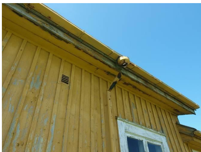
Fig. 2. Corroded and malfunctioning rainwater pipe
