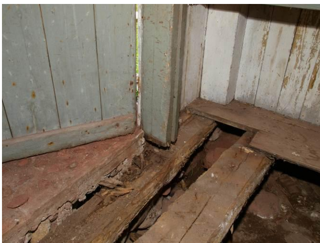
Fig. 17. Old fungal damage in room No. 3
