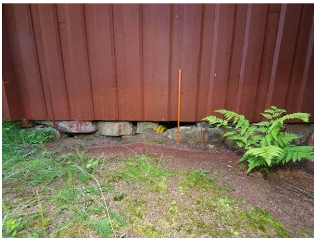
Fig. 2. The socket is too low and mortar between quarrystones is missing
