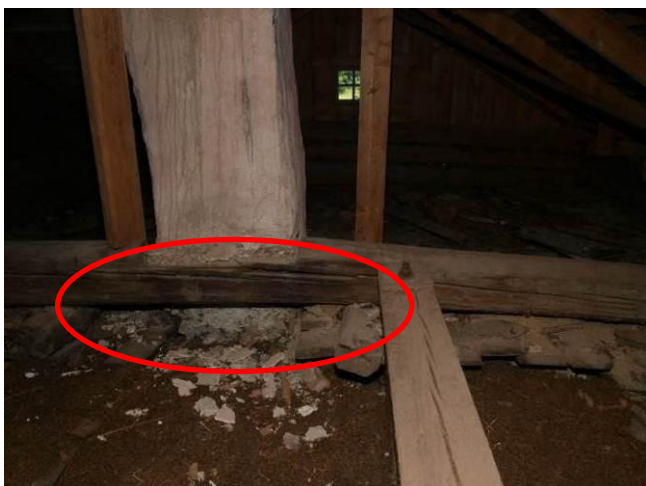
Fig. 13. The ceiling-beam has signs of losing its strength (cracks in tensile zone)
