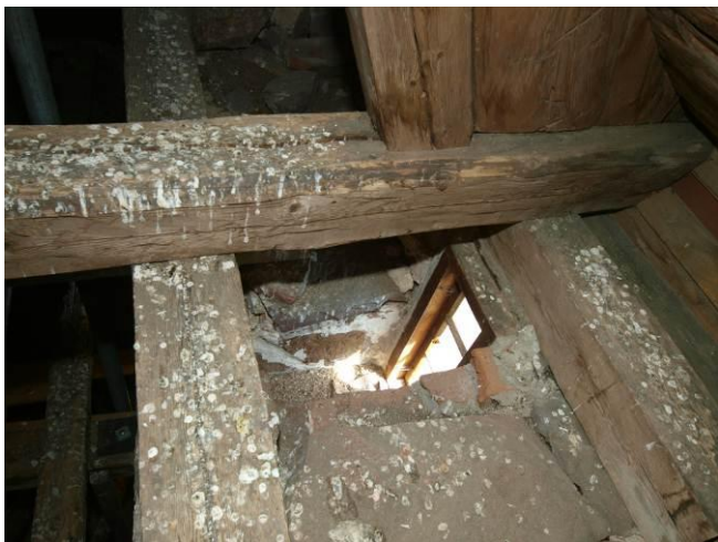
Fig. 4. Timber elements covered with birds' excrements.
