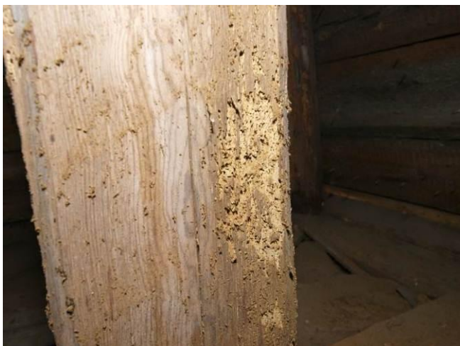
Fig. 5. Beetle attack on the beam
