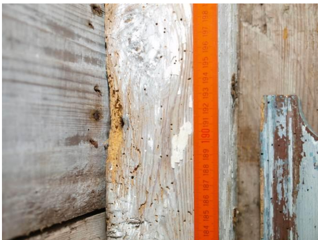
Fig. 7. Exit holes of the common furniture beetle on the wall
