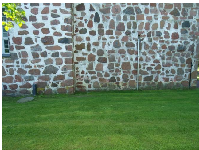
Fig. 2. Biodamages on the walls near the ground
