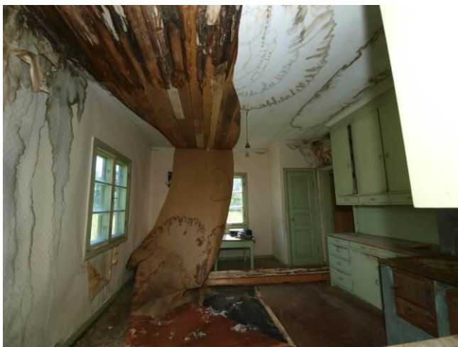
Fig. 19. Severe water damages in the kitchen
