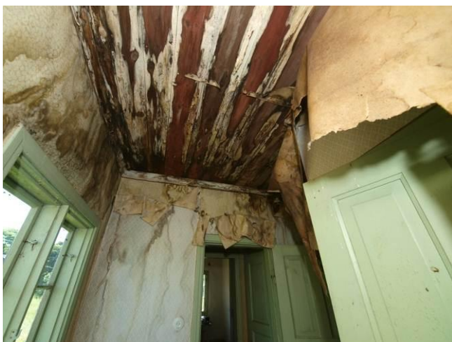
Fig.32. Fungal attack on the hall ceiling
