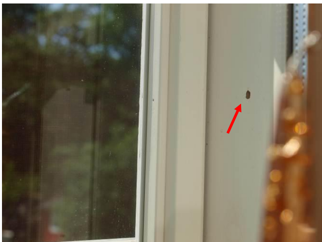
Fig. 10. Exit hole of the Old House Borer in the window frame
