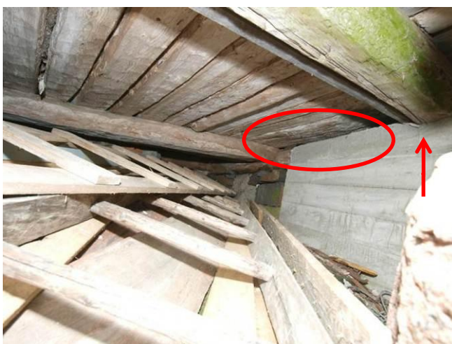
Fig. 6. Missing hydro-insulation between the bearing floorbeams and stone foundation
