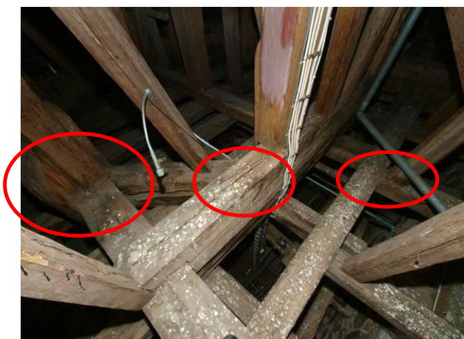
Fig. 6. Traces of old water damages and timber elements covered with birds' excrements
