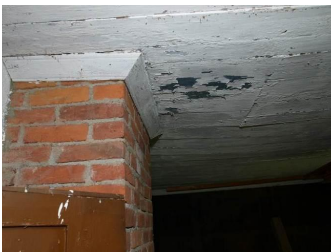
Fig. 10. Peeling paint from the ceiling in room No. 8
