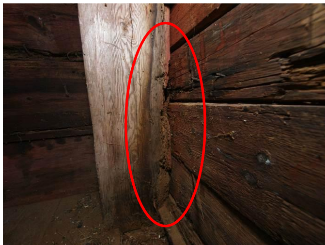
Fig. 8. Massive beetle attack on the beam
