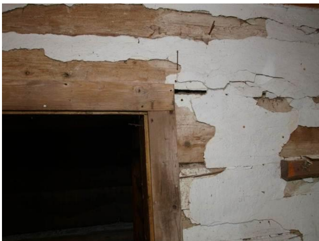
Fig. 8. Loose and missing plaster on the wall in room No. 6
