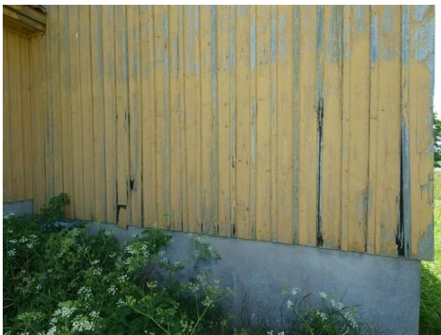
Fig. 5. The wall boarding has partially degraded and paint has flaked off
