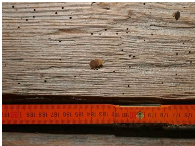
Fig. 12. Exit holes of anobiid beetles
