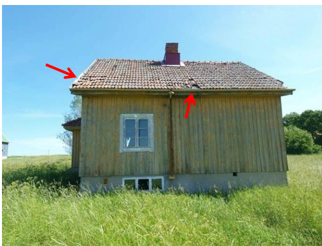
Fig. 7. Some roofing tiles are missing and broken on the western side
