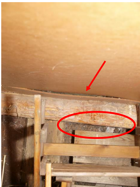
Fig. 5. Missing hydro-insulation and there are gaps in the ceiling's covering layers (in the basement)
