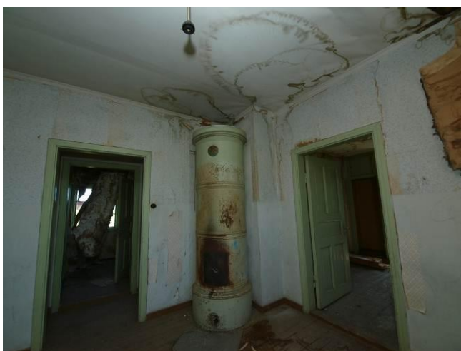
Fig. 24. Severe water damages in the livingroom
