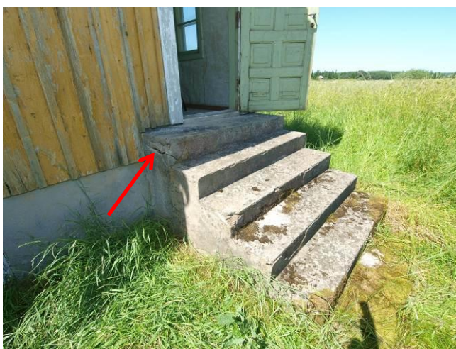
Fig. 4. Cracked and biodamaged staircase
