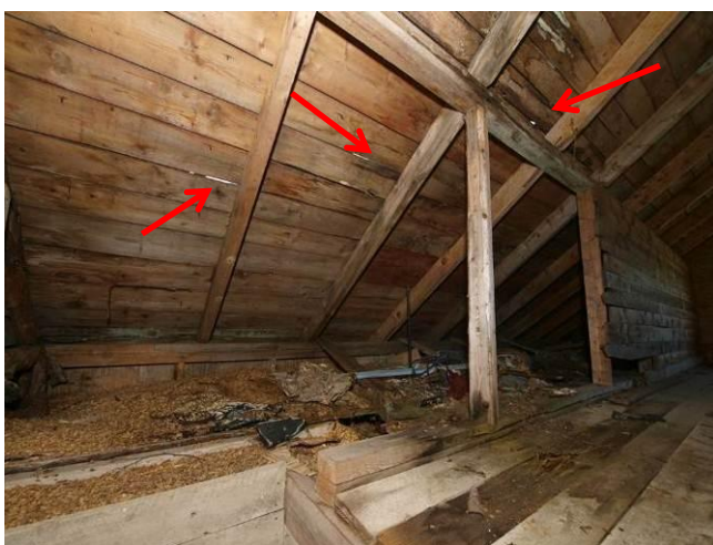
Fig. 26. Water leakages in the roof
