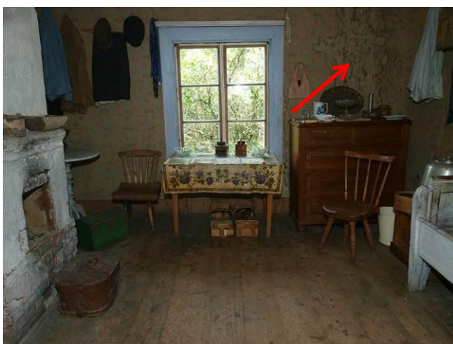
Fig. 9. Traces of water passage on the wall in the room No. 1
