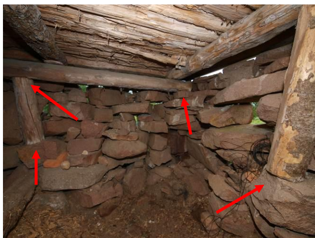
Fig. 4. Missing hydro-insulation, unstable timber joints
