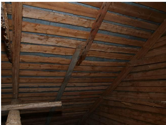
Fig. 10. The gap between the rafters is too big, a risk of hogging of barks
