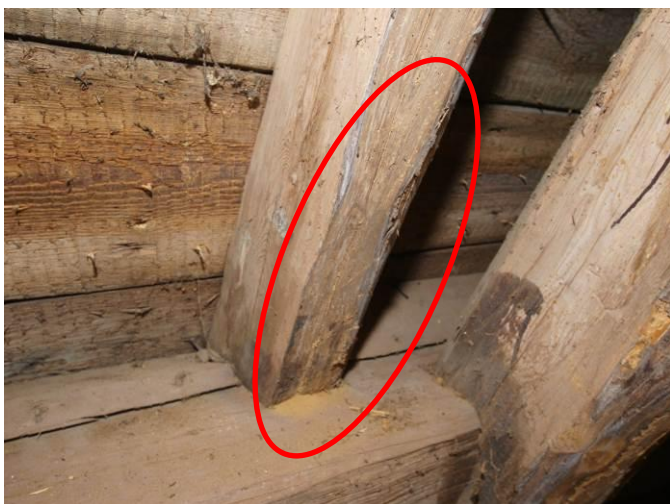
Fig. 4. Bore dust and exit holes on the timber construction
