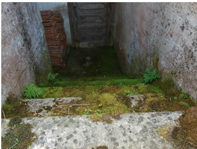
Fig. 9. The cellar's stairway has no hatch, causing severe water load down to the basement. The stair steps and floor are covered mostly with mosses
