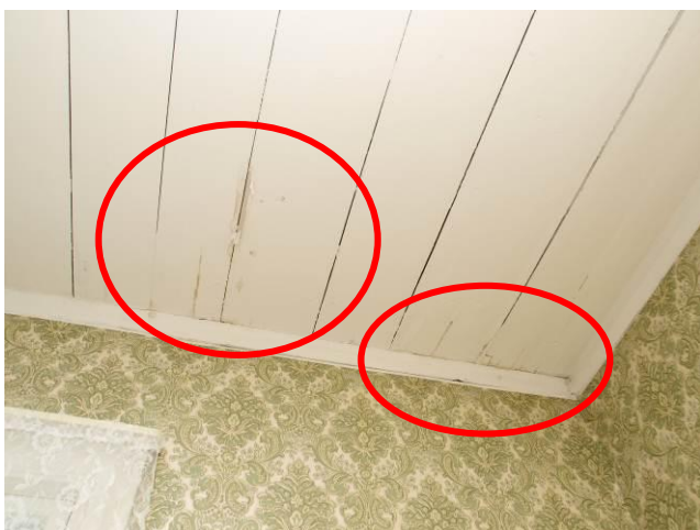
Fig. 6. Traces of water passages
