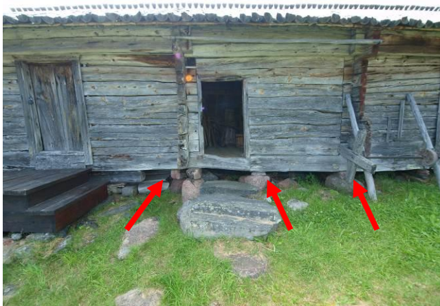
Fig.1. Missing hydro-insulation, hogged logs of the wall
