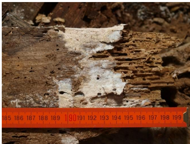
Fig.37. Fungal and beetle damages on the floorboards
