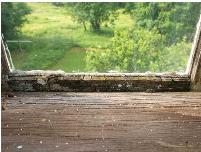
Fig.18. Lichens growth on the windowframe
