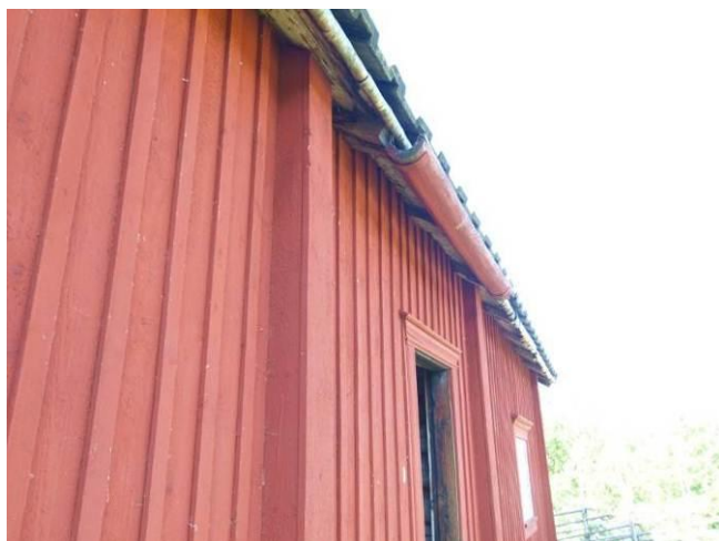
Fig. 1. The rainwater system is incomplete
