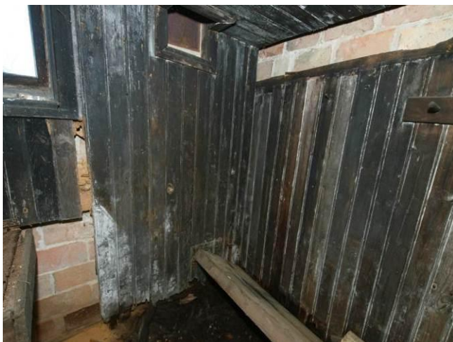
Fig. 14. Degraded timber elements in sauna
