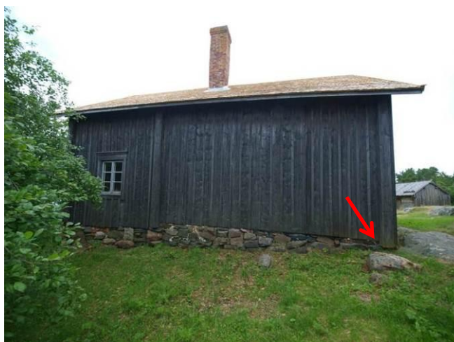
Fig. 2. Biodamages on the lower parts of the wall
