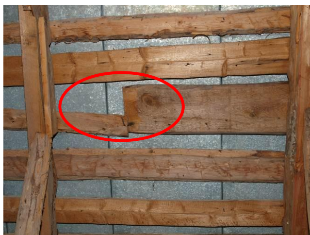
Fig. 11. Barks are spliced between the rafters
