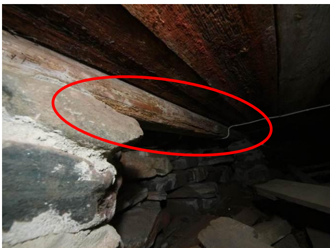
Fig. 11. Bearing floor beam attacked by beetles
