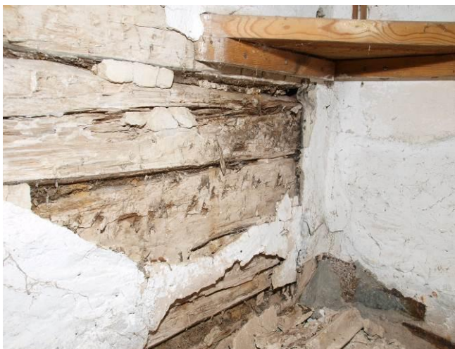
Fig. 16. Old fungal damages in room No. 6
