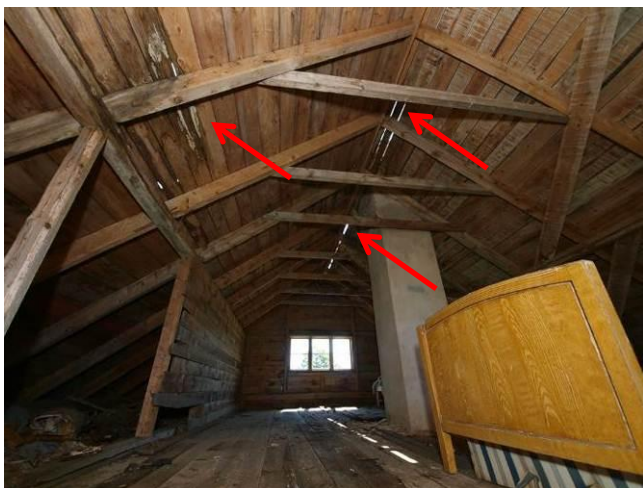
Fig. 25. Water leakages and degradation of timber elements in the roof structure
